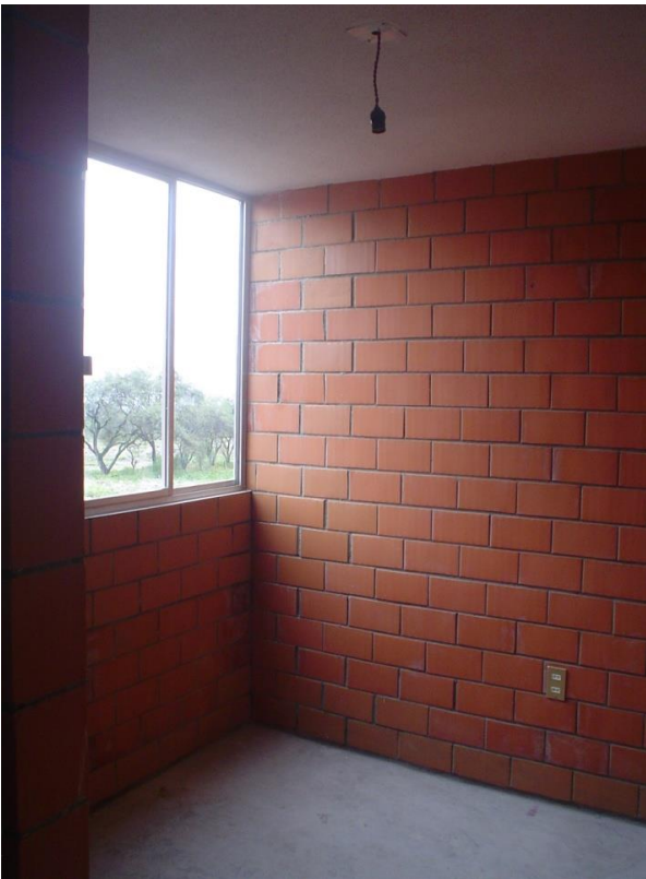
VISTA INTERIOR RECAMARA
